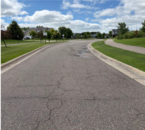
W. Lake Blvd and Woodland Pkwy
