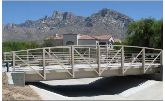
Big R Pedestrian Rolled Girder Bridge
