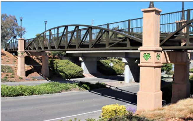
Continental Pedestrian Truss Bridge
