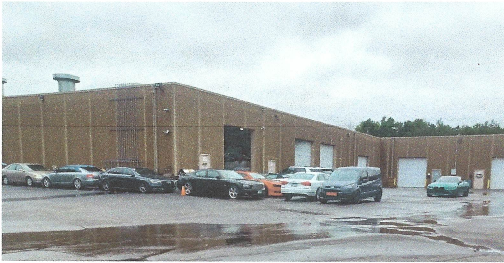
Notice customer cars are being stacked outward into courtyard. The unit with the open garage door is 307 and 306 is next to it with gray floor paint on the upper corner.
