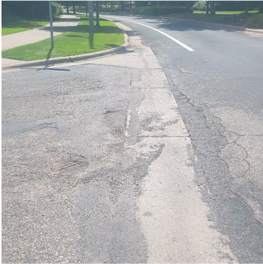
Figure 2-1 Existing Conditions South Lake Blvd NE at 119 th Ave NE (looking south)
