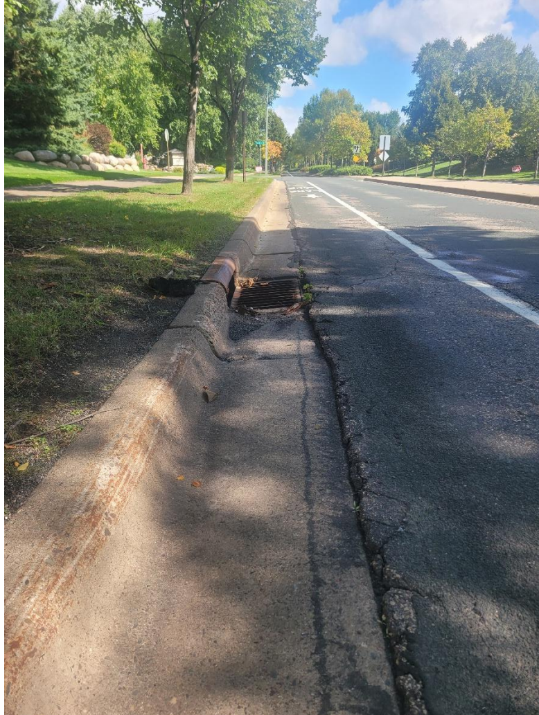
Figure 2-4 Existing Conditions South Lake Blvd NE at Dunkirk Circle NE (looking north)
