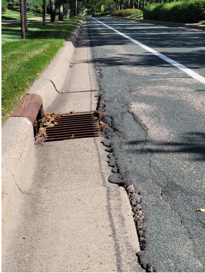
Figure 2-3 Existing Conditions South Lake Blvd NE at Flanders Circle NE (looking north)
