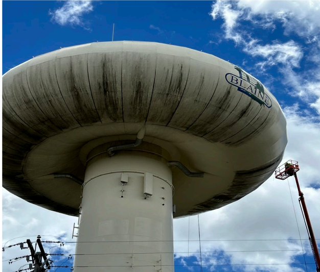
Completed in May Tower #1 Cleaning
