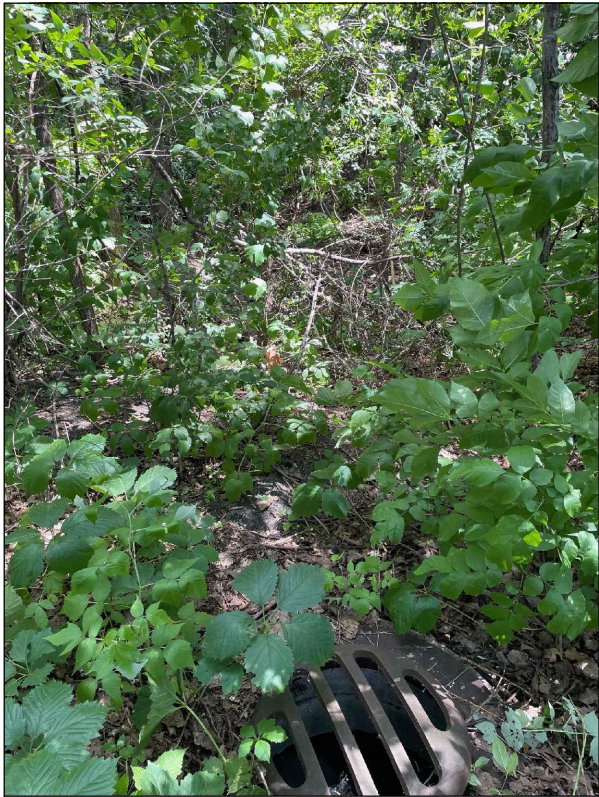
LOOKING EAST AT EX. CBMH 101
