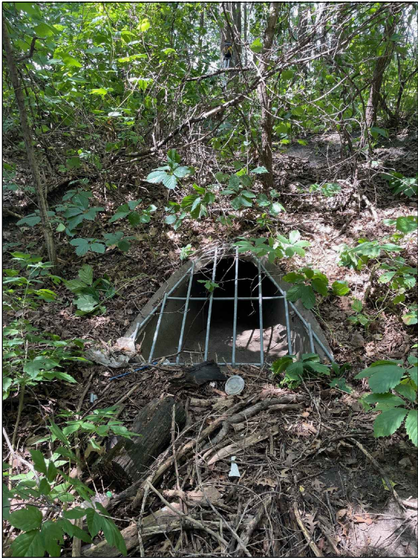
LOOKING WEST AT EX. FES 2
