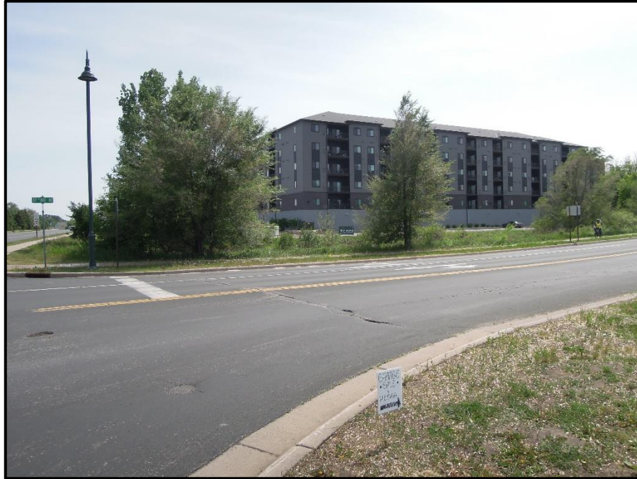
Looking South towards Subject from Intersection of 117 th Ave. NE & Ulysses St. NE
