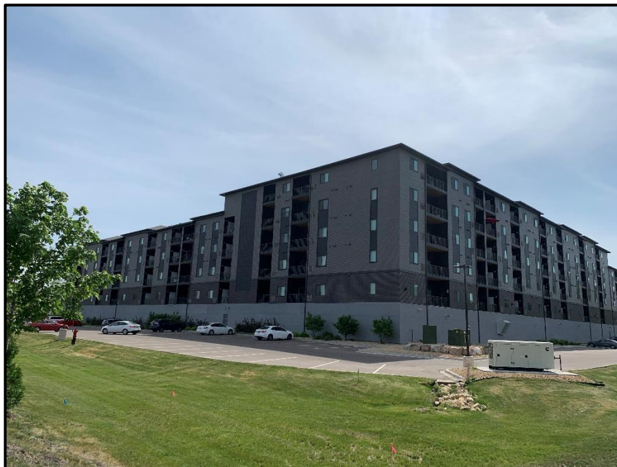
Looking Southwest at Subject Building Improvement
