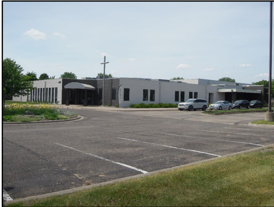
Looking Northwest at Artisan Church's Building Improvement
